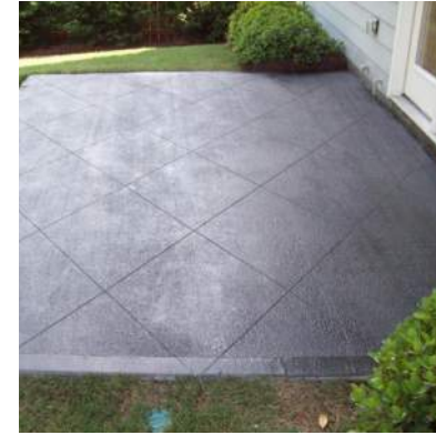
Scored concrete driveway doubles as patio
