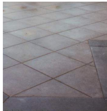
Scored concrete paving
