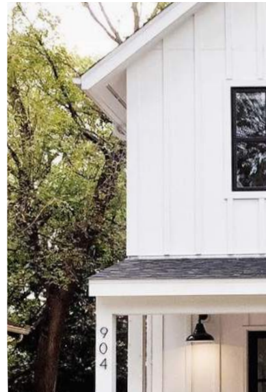
Overhanging roof eaves
